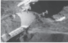
The Hoover Dam is a 221-metre high concrete arch-gravity dam in the Black Canyon of the Colorado River in the United States of America. It was built to provide irrigation water, to control floods, and to provide water for a hydroelectric power station at the base of the dam. Figure 1: Hoover Dam Figure 2: The site proposed for the dam in about 1921. Figure 3: A sketch of the proposed reservoir. Figure 4: Plans Figure 5: Plans
